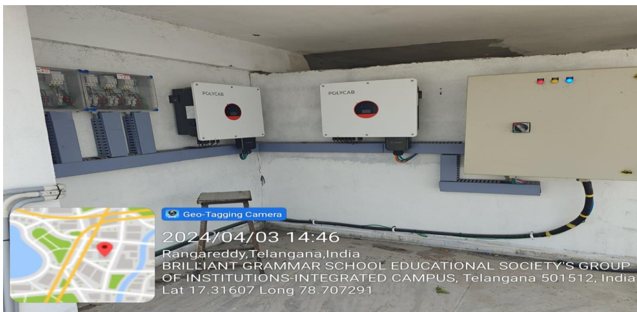
Wheeling to GRID connection.
